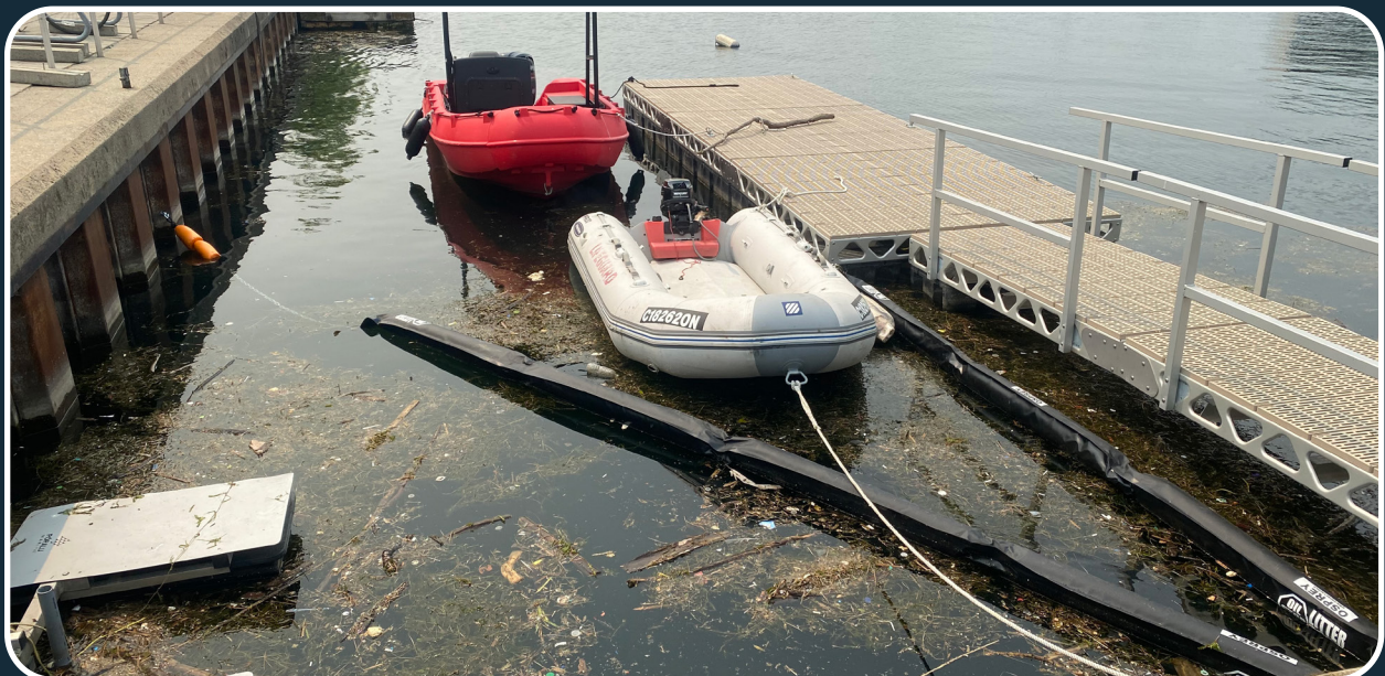
Trash capture devices, including the litter boom and Seabin pictured above, were installed at three sites in the Toronto harbour: Peter Street Basin, Police Basin, and Marina Four/Simcoe Wave Deck. Source: Osprey Initiative
