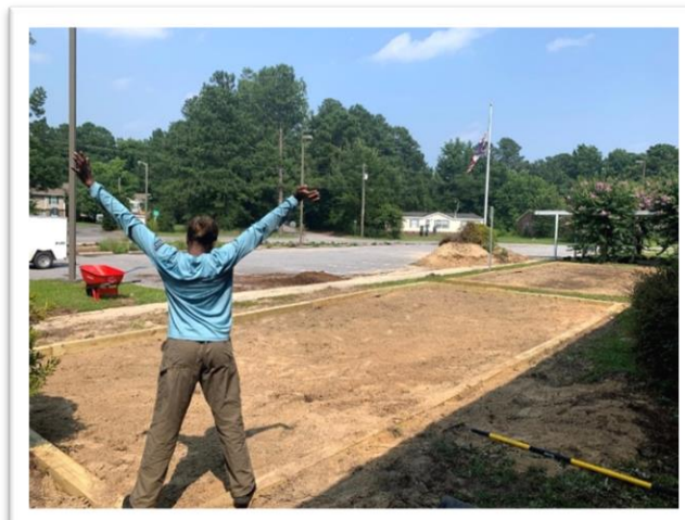
Figure 3: Crew members building a rain garden for stormwater capture.
